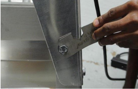
Use the Zeco® wrench provided to tighten the bolts
